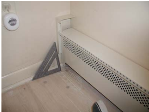
#1 – Position face panel. Slide end cap down to rest on top edge of base molding.
