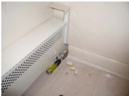
#5 – Completely chisel out base molding notch.
