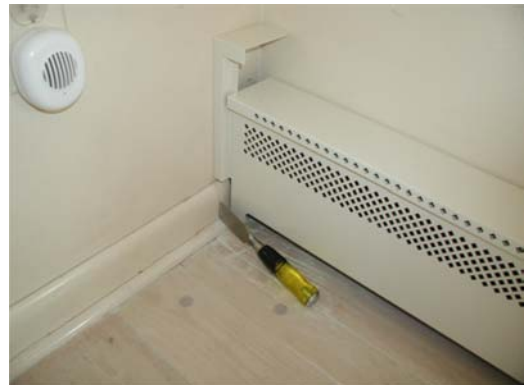
#4 – Use sharp chisel with wide blade to carefully notch base molding (or Dremel).
