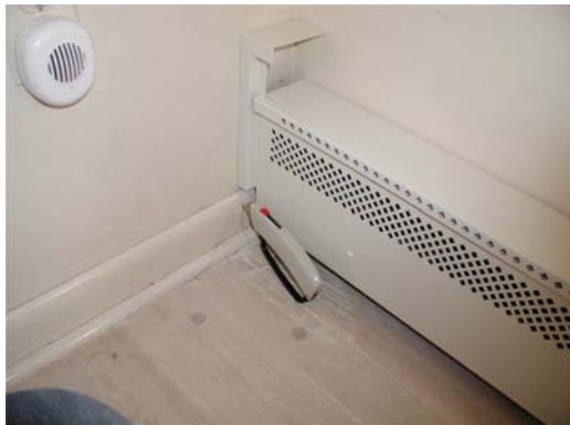
#3 – Scribe notch line with utility knife to score notch line.
