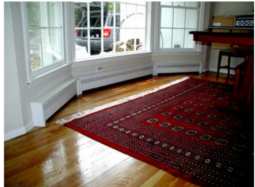
#6 – A finished non-90 degree corner. Please allow 30-days for Radiant Wraps to fabricate the custom top rail wedge piece.
