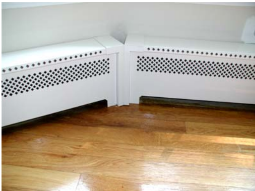
#5 – Once the corner joint is created, a template of rigid cardboard must be provided to Radiant Wraps for us to make the custom top rail wedge piece.
