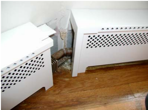
#3 – The right open end cap will be installed.
