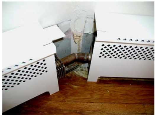
#2 – The positioning of the two intersecting panels (determined by the measuring gauge) will allow for the left and right open end caps to create the new corner.
