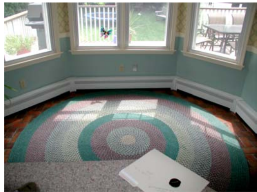
#4 – This picture shows the finished bay window with multiple top rail wedge pieces.
