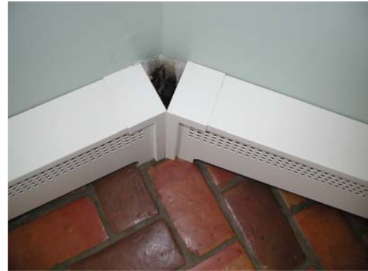
#2 – This photo shows the two adjoining panels in place with left and right open end caps. You are now ready to install the top rail wedge piece that will cover this opening.
