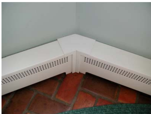
#3 – The top rail wedge piece is custom-made as per the customer-provided template described in the Bay Window Measuring Instructions page. The wedge piece will be secured with two dabs of adhesive caulk. This will allow for easy removal in the event that access is needed to the heating element fins.
