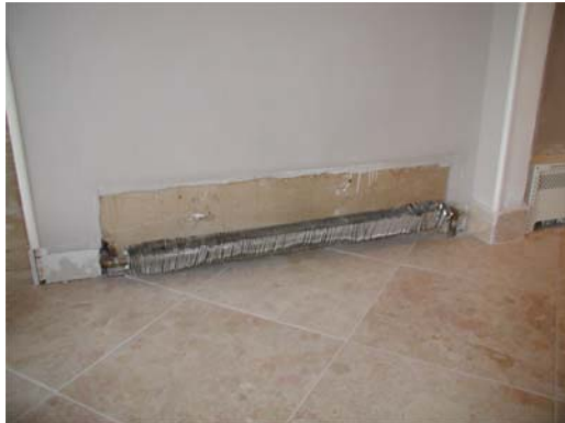
#1 – Mounting brackets used for install when back panel of enclosure is missing.
