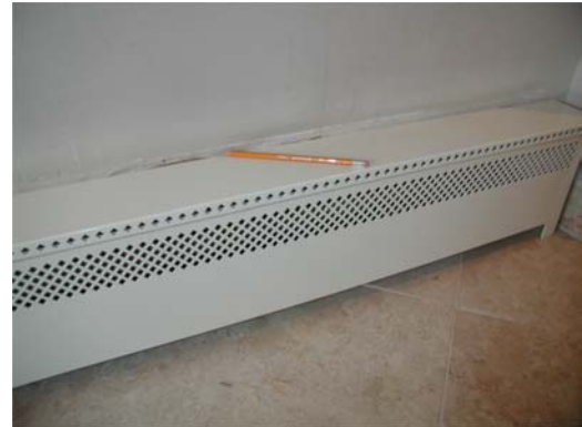
#2 – Position panel and lightly mark height of top rail on the wall. Tip panel forward and mark the location of the back teeth.
