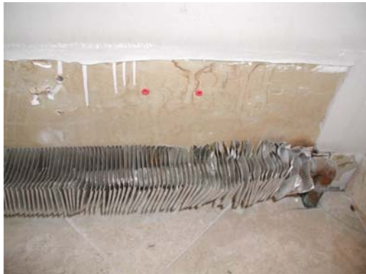
#3 – Position mounting bracket 1/8" below top line and in between teeth. Pre-drill and install plastic anchors when there's no stud.
