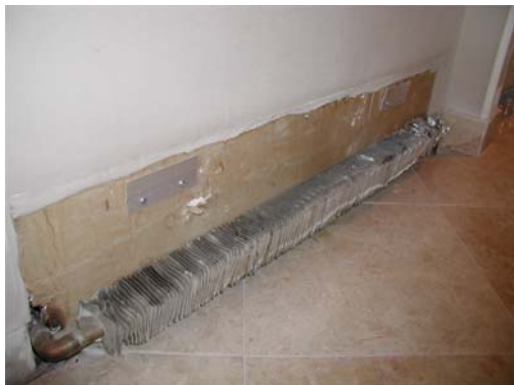
#5 – Install two mounting brackets for each panel.
