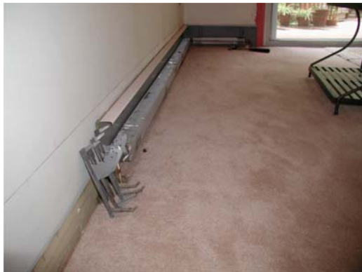
#3 – Slide all existing support brackets out from existing back panel.
