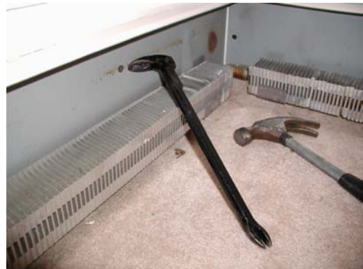
#4 – Remove existing nails or screws that anchor the back panel to the wall.
