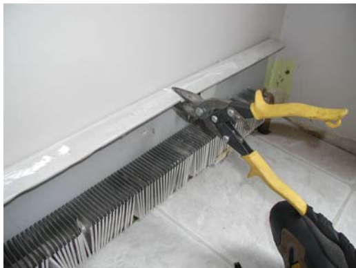
#1 – Use metal snips and slice top rail from front to back. Be careful of sharp edges.
