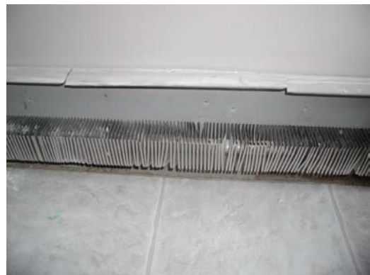
#2 – Slice top rail into 10" to 12" sections.
