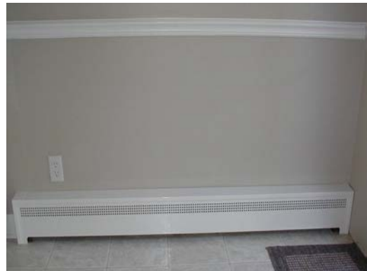
#6 – Slide new panel down into place.
