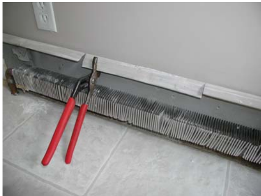
#3 – Using a heavy set of pliers, bend down each 10" to 12" section.
