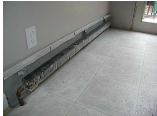
#4 – Bend down entire top rail across the length of the back panel.
