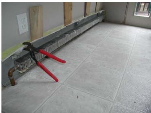
#5 – Slide shims behind back panel and make final bend down to desired height.
