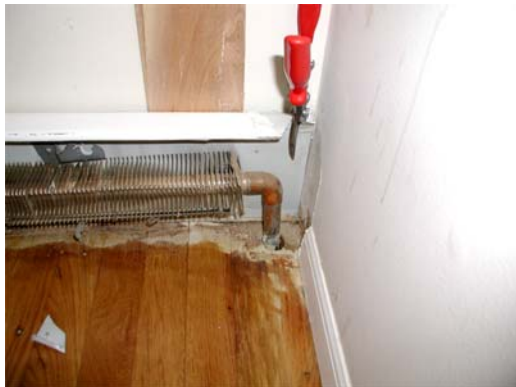
#3 – Carefully snip out \frac{1}{4} " to \frac{1}{2} " of back panel from top to bottom or use open end caps that require a smaller notch.
