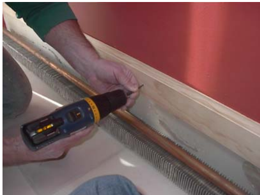
#3 – Install tin flashing and spacer board to the wall.
