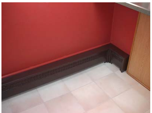
#6 – Install new Radiant Wraps panels onto mounting brackets.
