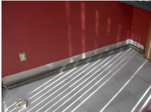
#1 – Remove existing back panel of enclosure to prepare for spacer board and flashing installation.
