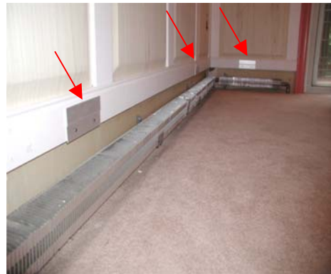
#4 – Mounting brackets installed to base molding.
