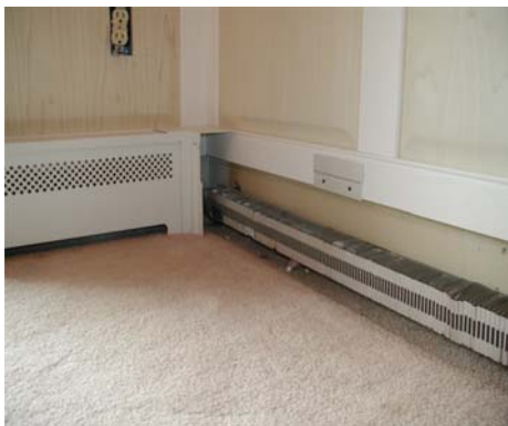
#5 – Installation partially complete to inside corner.
